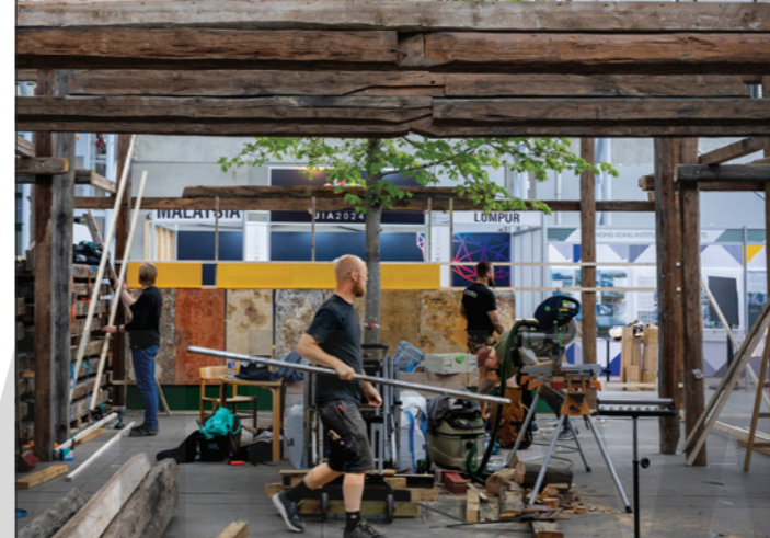
The construction wood for the pavilion came from The Red Storage Building, done by architect N. S. Nebelong in 1883; it was sourced by the Danish company Genbyg—the largest online webshop in Denmark for reused building materials—that provided all wood for the pavilion
